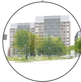
Two new floors on top of existing towers. New winter gardens to existing 1 bed flats
