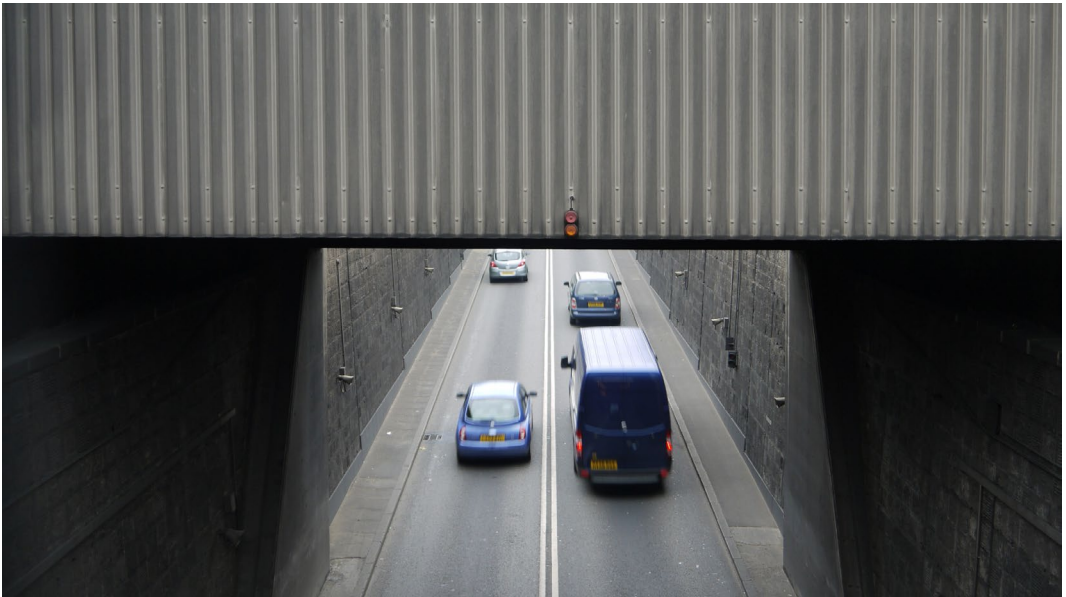
Figure 16 Blackwall Tunnel, south exit.
