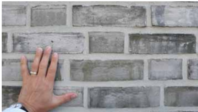
Fig 5.7.1 Waterstruck bricks have a softer appearance and work well adjacent to older build-
